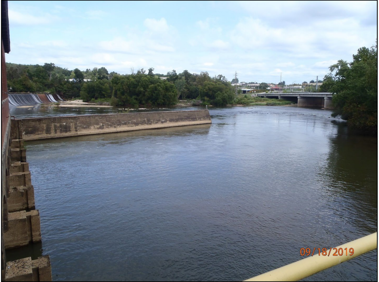
Figure 1.8.6-1. Photograph of the Project tailrace.
