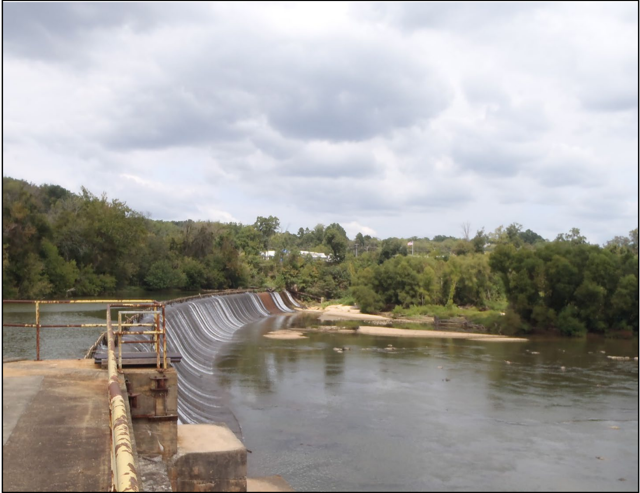
Figure 1.8.1-1. Photograph of the Project dam.
