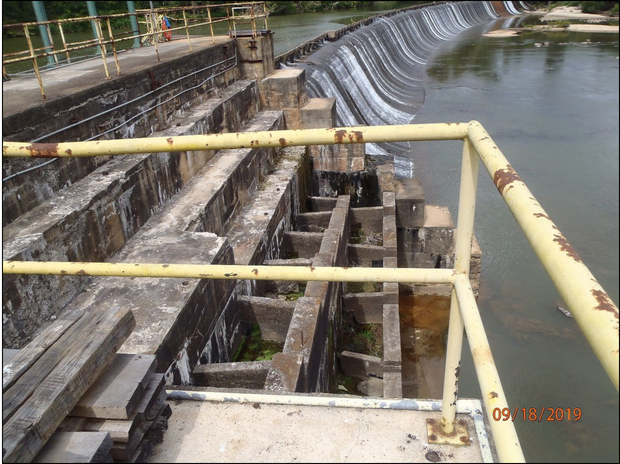
Figure 1.8.4-1. Photograph of the Project headwall section.
