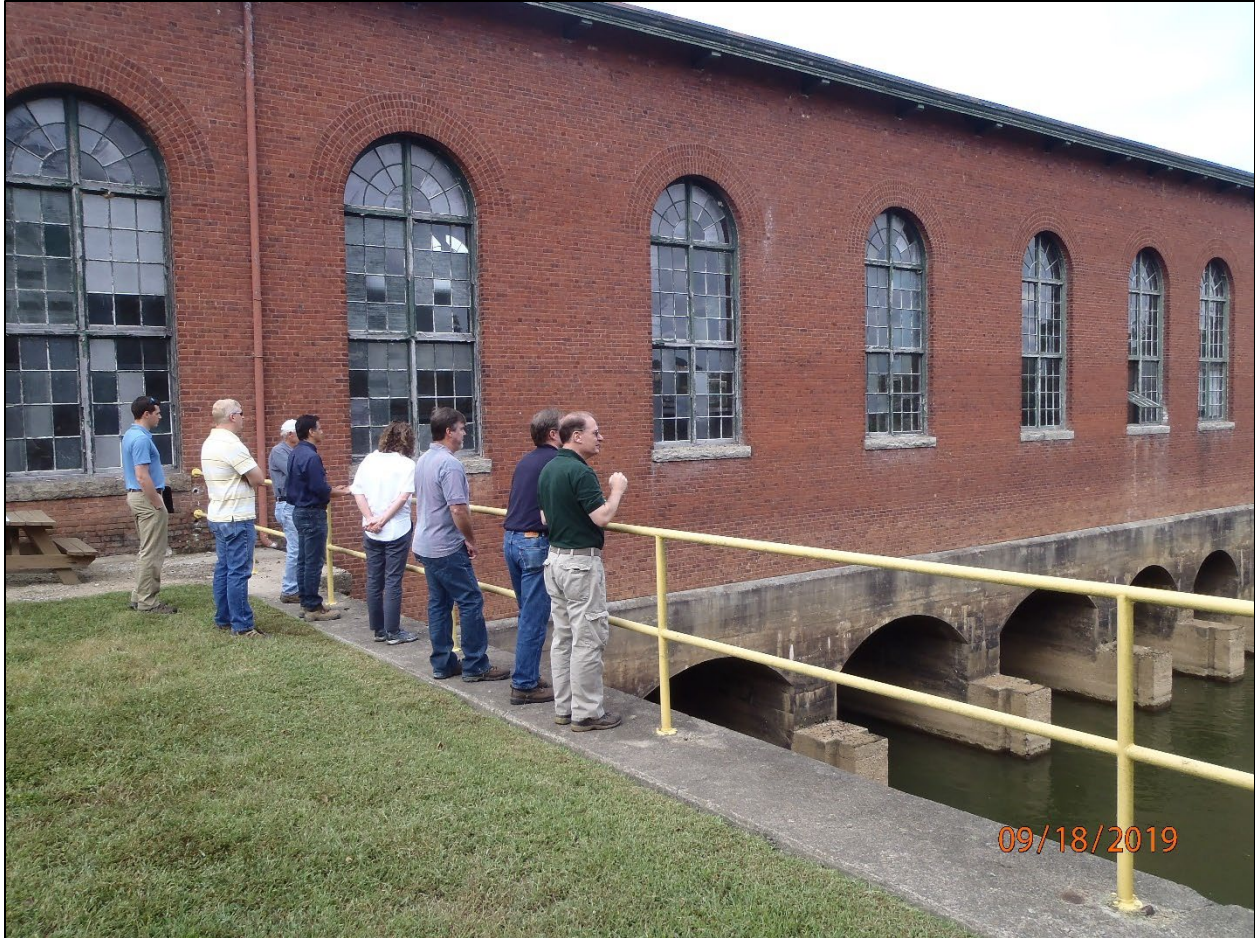
Figure 1.8.5-1. Photograph of the Project powerhouse exterior.
